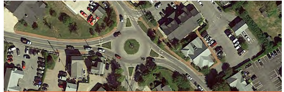
NANTUCKET, SPARKS AVENUE/HOOPER FARM ROAD ROUNDABOUT NEAR FIRE STATION
